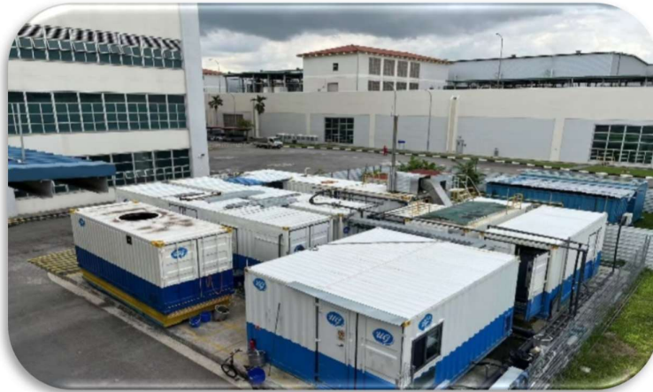
Sludge Treatment System housed in containerised modules at Changi Water Reclamation Plant
